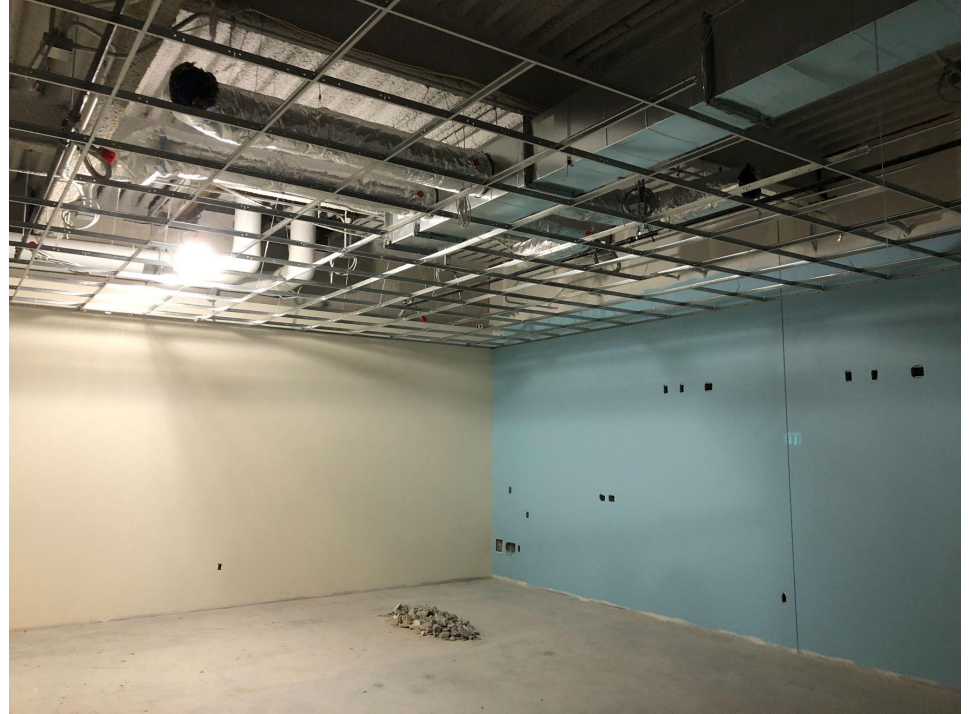
Painting and Ceiling Grid Install
