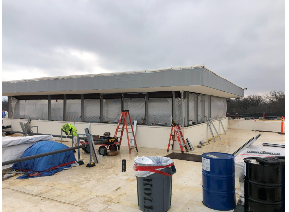
Clerestory Installation at South Vestibule/Tower
