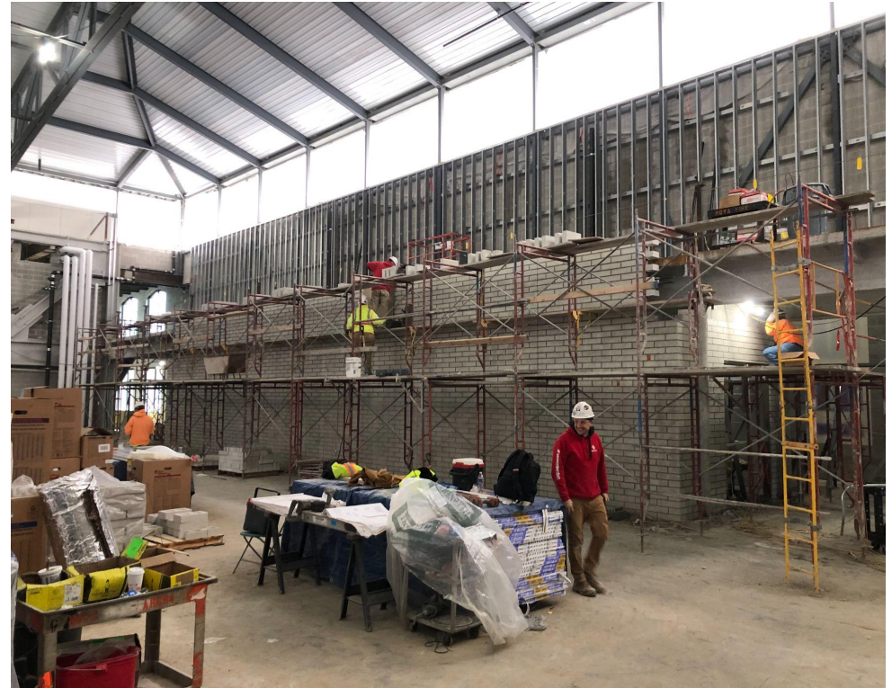
Ground Face CMU being install in Comp. Gym
